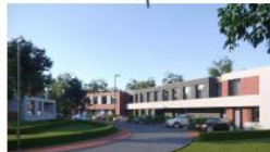
Row House (9 sections) Construction Q3.2018.-Q3.2019.
