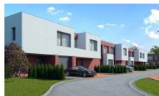
Row House (7 sections) Construction Q4.2017.-Q4.2018.
