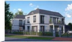
Twin Villa Camellia Construction started—till Q2.2018.
