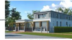
Villa Helena Construction started—till Q2.2018.
