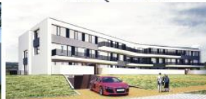
Apartment House (27 apartments) Construction Q3.2018.-Q3.2019.
