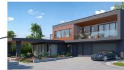
Villa Lavanda Construction started—till Q2.2018.
