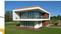
Villa Corylus Construction finished.
