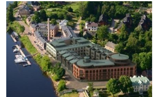
Unique riverside apartment building complex 'Gypsum Factory'
