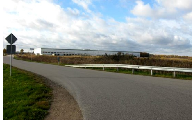
/Paved site access roads/
